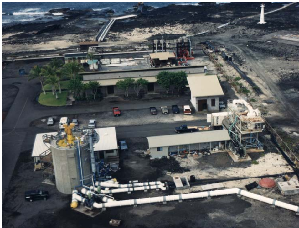
Figure 8 210-Kilowatt Open-Cycle Ocean Thermal Energy Conversion Experimental Apparatus
