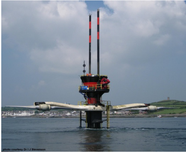
SeaGen twin turbines with two 16-meter diameter rotors shown above water
