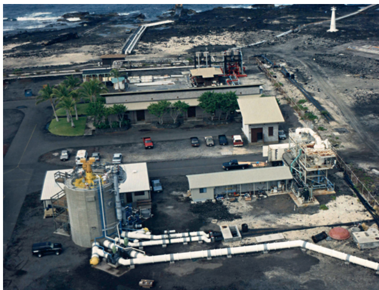
Ocean Thermal Energy Conversion. Figure 1 210 kW OC-OTEC experimental apparatus (1993–1998)
