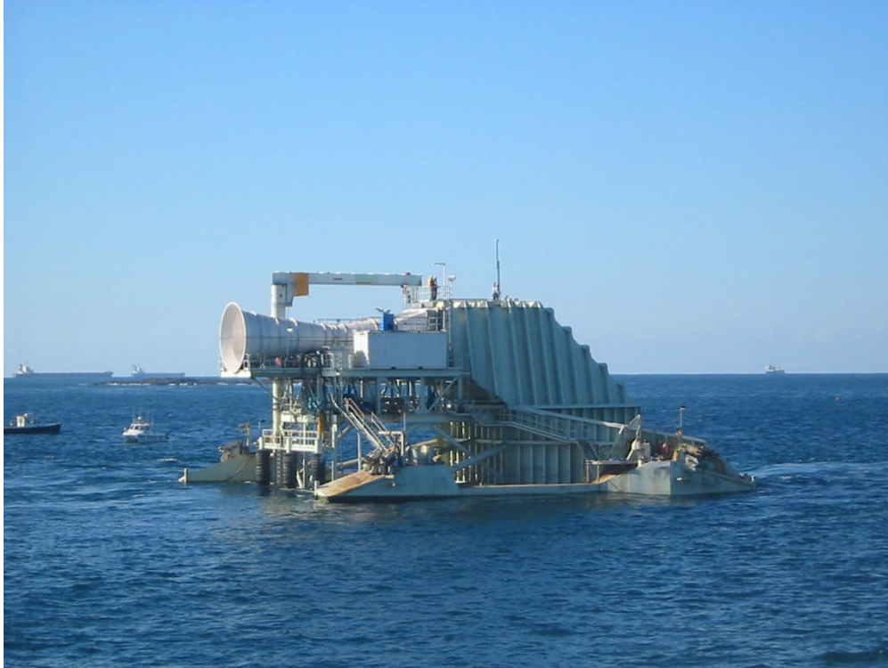
Oceanlinx Wave Energy Systems 97
